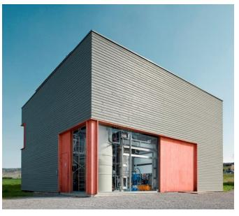
Smart Cities: In DEUS 21 project rain water is collected and processed in a central, modern membrane system to drinking water quality.
