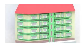
Building Systems: Heat recovery via a ventilation channel track in the facade of an apartment building with a minimally invasive restoration solution by prefabricated windows and insulation elements in a composite thermal insulation system. © Fraunhofer ISE
